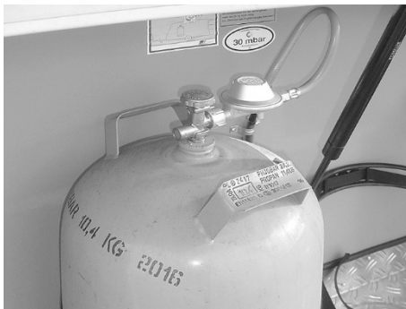
Fig. 112: Gas bottle with pressure reducing valve
