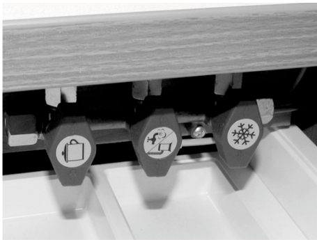
Fig. 91: Quick-closing valves
