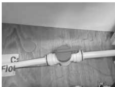
Fig. 86: ALDE floor heating valve
