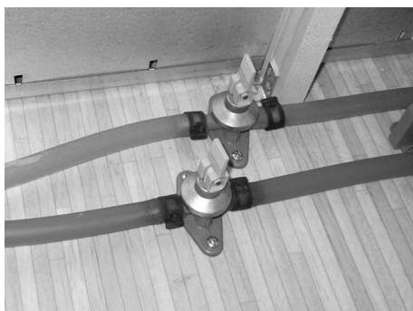
Fig. 97: Drain valves opened
