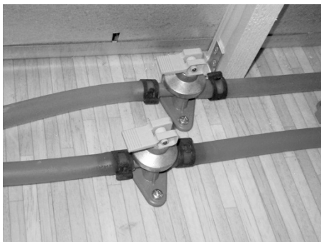
Fig. 171: Closed drain valves
