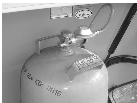
Fig. 94: Gas bottle with pressure reducing valve
