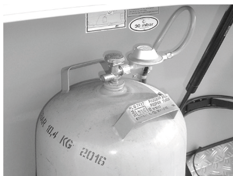
Fig. 74: Gas bottle with low pressure regulator and low pressure hose
