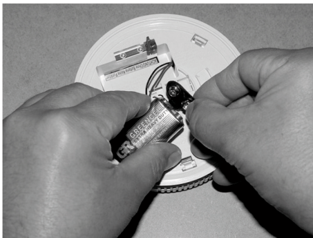
Fig. 202: Replacing the block battery
