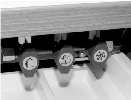
Fig. 80: Quick-closing valves
