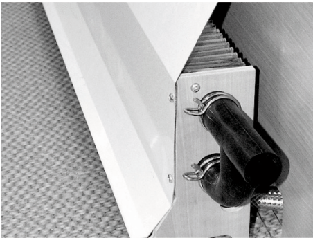
Fig. 89: Convector with thermally conductive panel
