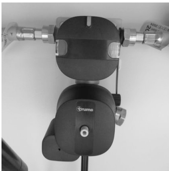
Fig. 112: DuoControl CS gas supply
