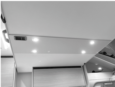
Fig. 58: LED spotlights below the lift-up bed
