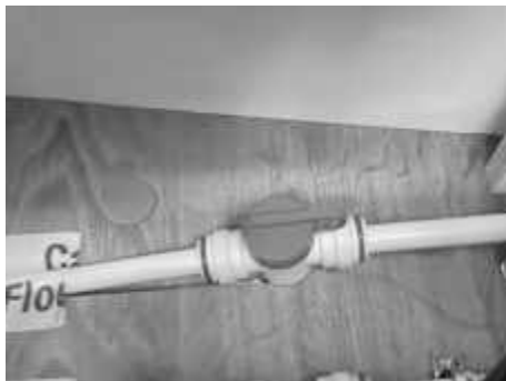
Fig. 99: ALDE floor heating valve
