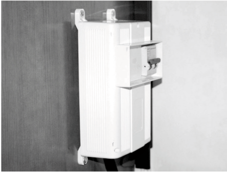
Fig. 66: Ground fault circuit interrupter (GFCI)
