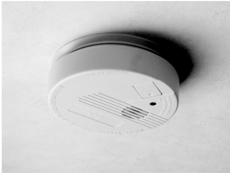
Fig. 50: Smoke detector
