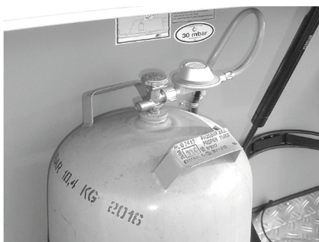
Fig. 81: Gas bottle with low pressure regulator and low pressure hose
